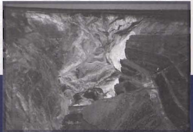
The visible effect of cave mining below an open pit on pit wall and surface stability
