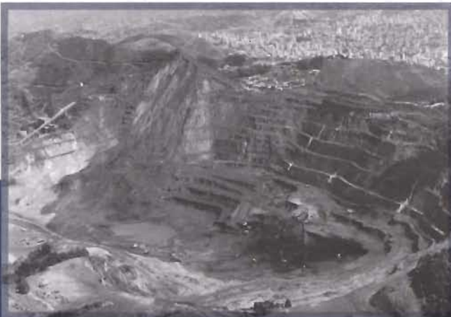
Patrimonio Landslide at the Aguas Claras Mine, Belo Horizonte (the city in the background), Brazil
